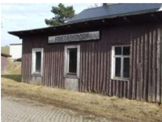
Abb. links: Wartehalle Friedersdorf
